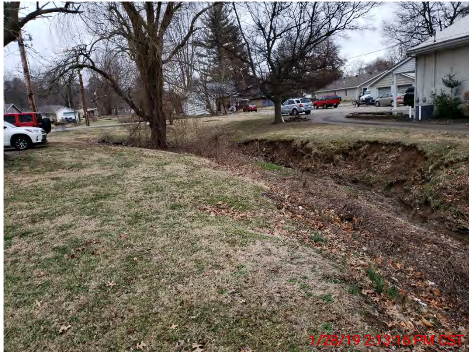
FIGURE 2-18 (AREA 5) ERODING BANKS ALONG DITCH AT 315 STATE STREET
