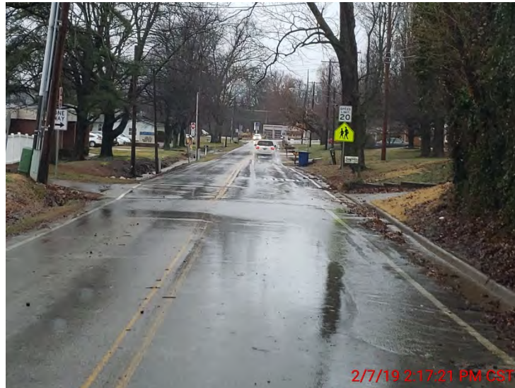
FIGURE 2-36 (AREA 11) SHEET FLOW ACROSS FRAME ROAD
