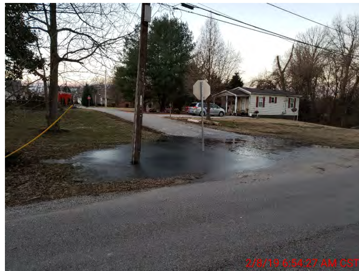
FIGURE 2-22 (AREA 6) 4 TH AND MONROE STREET SURFACE PONDING
