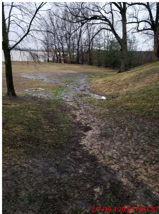
FIGURE 2-49 (AREA 15) WILLIAMS LANE PIPE OUTLET
