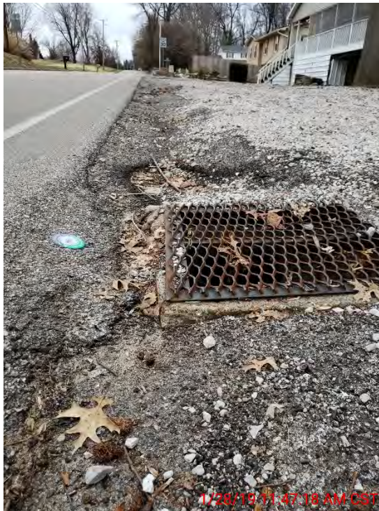
FIGURE 2-35 (AREA 11) INLET ALONG FRAME ROAD – NORTH OF VILLAGE LANE
