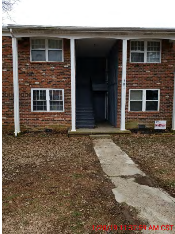
FIGURE 2-34 (AREA 10) LOW AREA EXPERIENCING PONDING ON VILLAGE LANE
