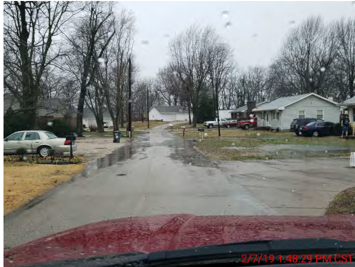
FIGURE 2-48 (AREA 15) WILLIAMS LANE PONDING IN YARDS AND ROAD
