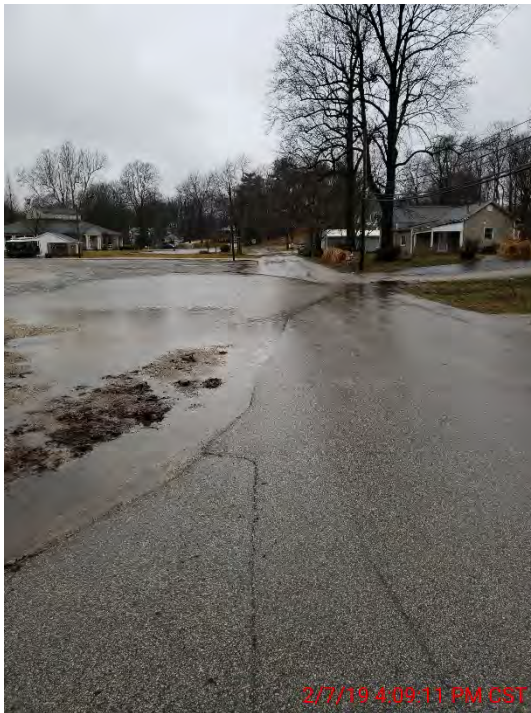
FIGURE 2-24 (AREA 6) PONDING AT THIRD STREET
