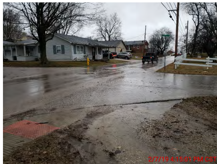
FIGURE 2-32 (AREA 9) STORMWATER SHEET FLOWS DOWN JEFFERSON AND POSEY STREET
