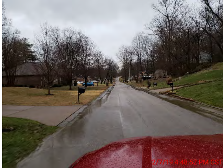
FIGURE 2-12 (AREA 2) CONCENTRATED FLOW ALONG EDGE OF PAVEMENT
