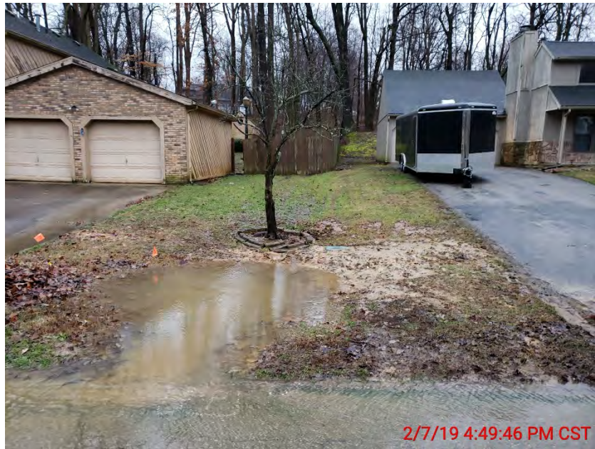
FIGURE 2-10 (AREA 2) PONDING IN RESIDENTIAL LAWN
