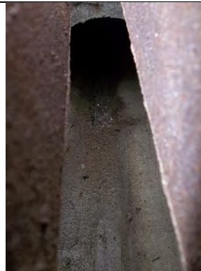
Interior Str. Looking at 12" RCP
