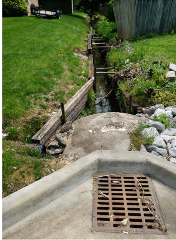
Figure 1: Forest Park Drive Culvert looking Downstream
