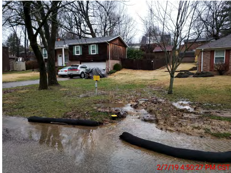
FIGURE 2-9 (AREA 2) PIPE REDUCTION SURCHARGE BOIL
