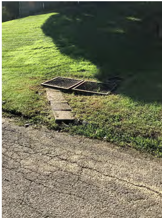
FIGURE 2-11 (AREA 2) INLETS ABOVE ROAD ELEVATION
