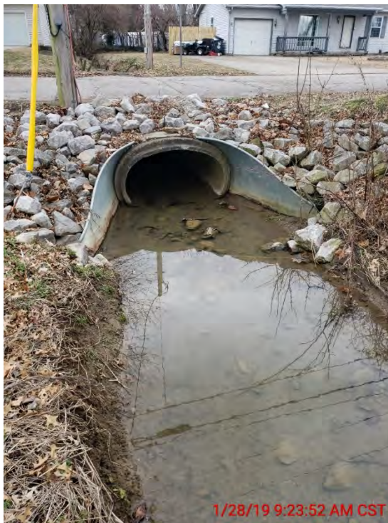
FIGURE 2-41 (AREA 12) MAPLE LANE 54" X 32" RCP CULVERT OUTLET
