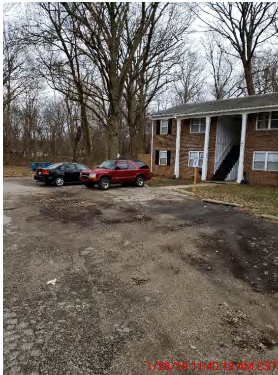
FIGURE 2-33 (AREA 10) LOW AREA EXPERIENCING PONDING ON VILLAGE LANE
