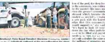
Newburgh Parks Board President Maryanne Whitehead (center) speaks to individuals gathered at the groundbreaking for the first phase of the Lou Dennis Community Park renovation project.
