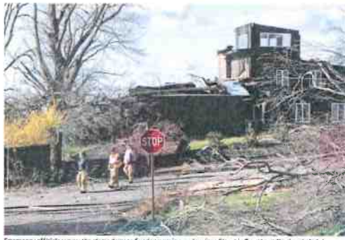
Emergency of Falls survey the storm damage Sunday morning on Jennings Street in downtown Newburgh, Ind. A tornado crossed the Ohio River from Kentucky and hit the area Saturday night. (COURIER PRESS FILE)
