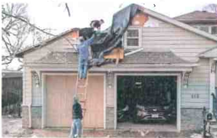
Venue Contracting workers John Mahesh, from top, Jeff Christian and Larry Riley nail a tarp over Mark Porter's garage Sunday on Jennings Street in Downtown Evansville. (COURIER & PRESS)
