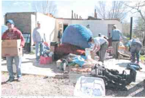
Friends, family and neighbors from Toyota Motor Manufacturing Indiana help the Mosleys repair damage to their home Saturday night in Newburgh, Ind. (COURIERPRESS.COM)
