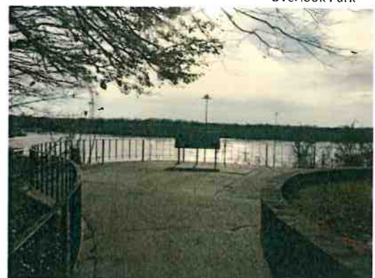
Figure 16 – Newburgh Locks Overlook in Overlook Park
