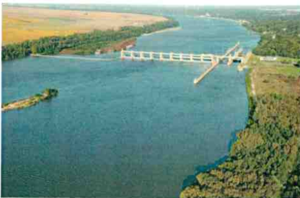
Figure 8: Newburgh Locks and Dam. lrl.usace.army.mil
