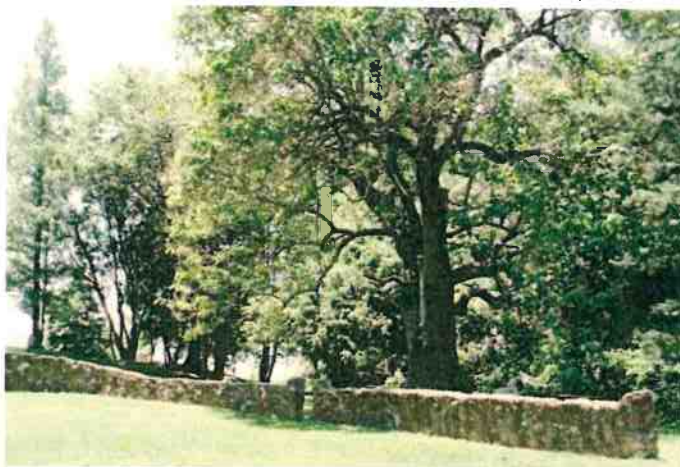
Figure 15 – Overlook Park Stone Wall
