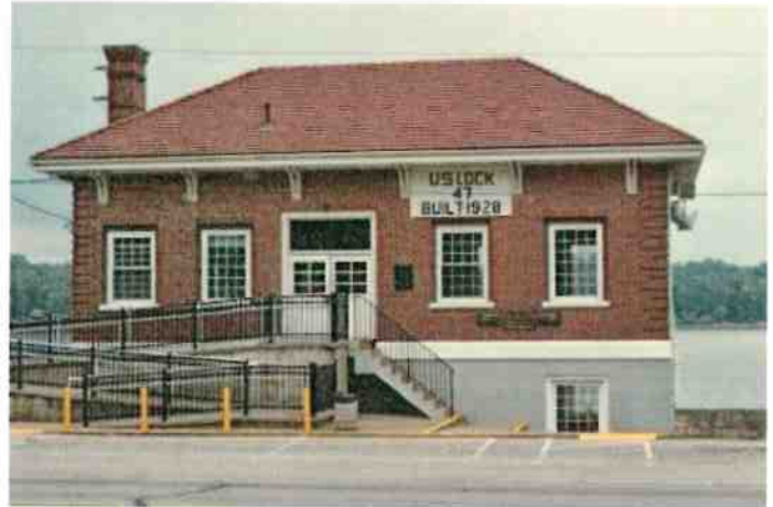
Figure 34 – Old Lock and Dam Control Building No. 47
