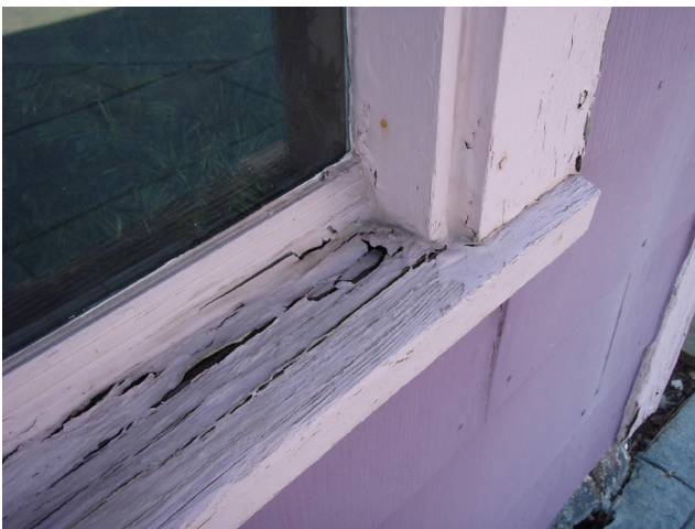
Check windows for peeling paint, rot (soft spots), caulk and glazing.
