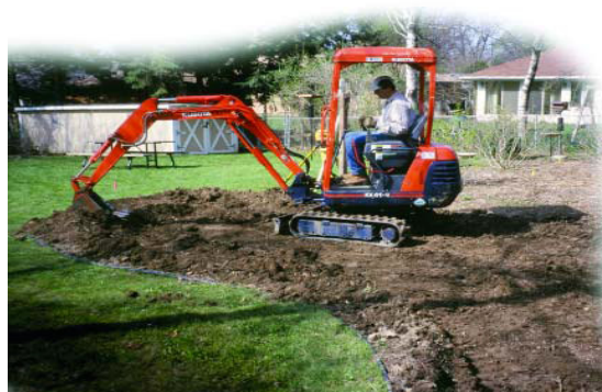
Digging with a rented backhoe.
