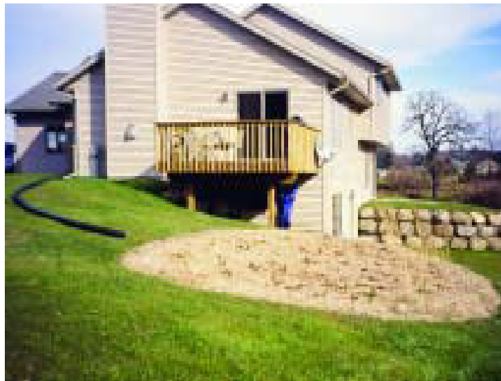
An extension of PVC pipe helps direct downspout water to this rain garden.
